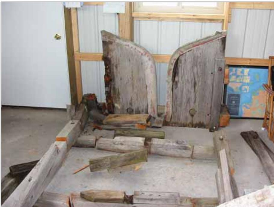
Enough of the cradle remained to permit taking measurements and to determine the wood required for reconstruction.
