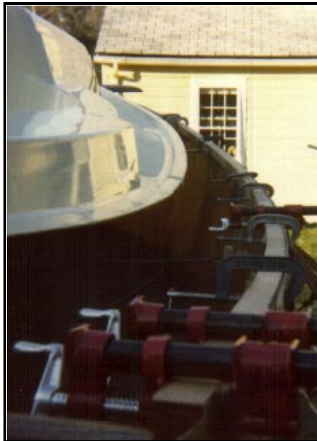
The sheer shelf was glued, screwed and clamped in place. The molded fiberglass lip on the deck fit right over this shelf.
