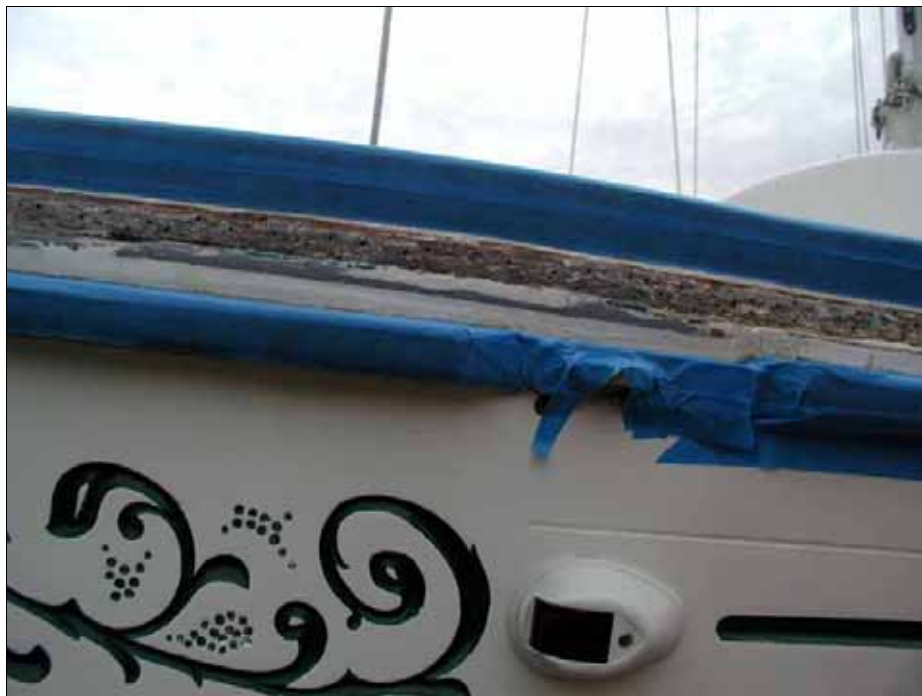
Another unexpected project. Fiberglass was missing over port bow area. Photo: Jim & Debbie Custer © 2005
