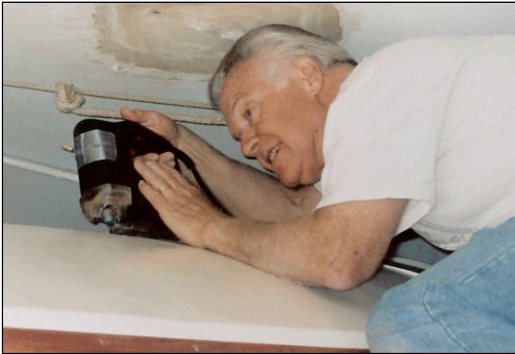
Cutting a hatch opening in tight conditions. Photo: Bob Collier© 2015
