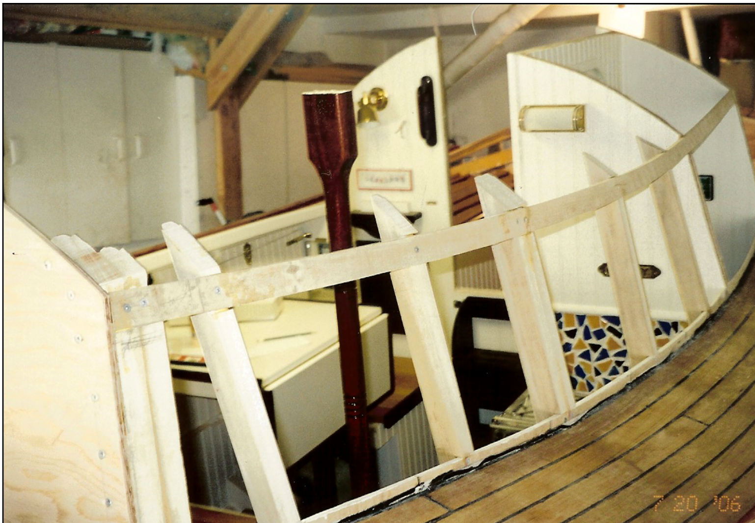
Getting ready for the coachroof to be installed. Photo: Bob Collier© 2015
