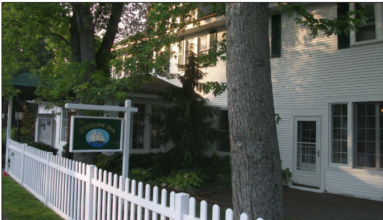
The Riverside Inn is one of many places in Leland that are from an earlier time. Photo: Randy Richardson © 2015
