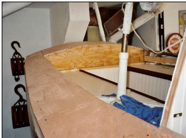
The beams were covered with plywood. Photo: Bob Collier © 2015
