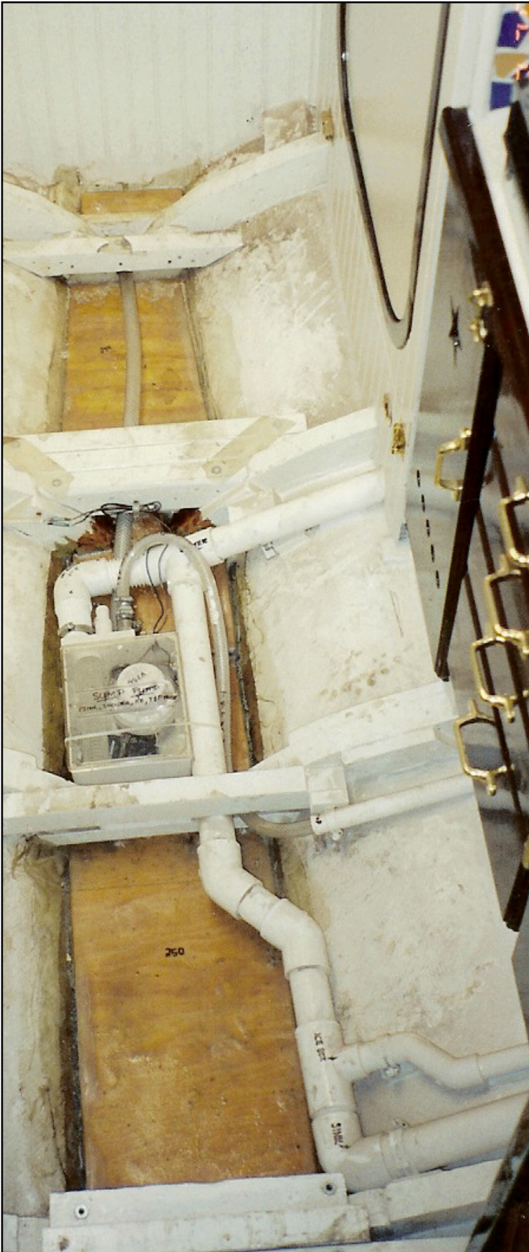
Photo 8: The plumbing system is complete! Photo: Bob Collier © 2014
