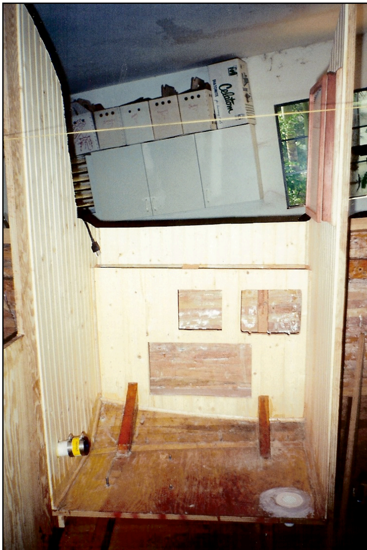
Photo 4: Roughed in head compartment. Photo: Bob Collier © 2014
