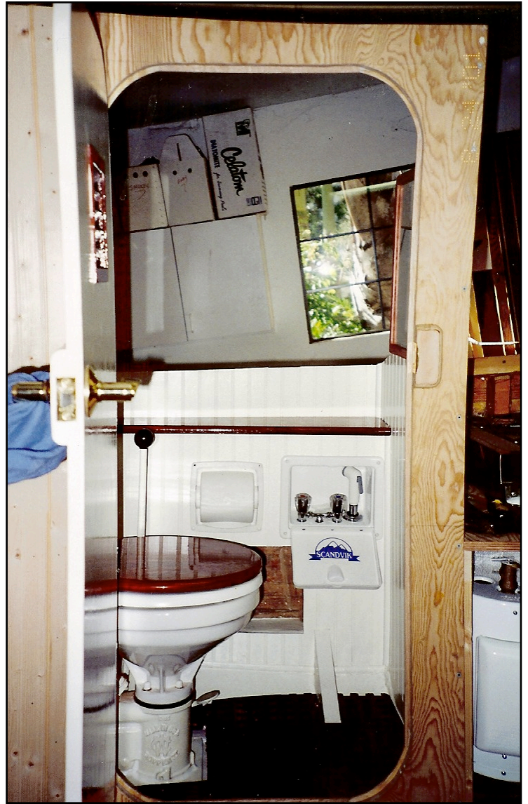
Photo 7: The head and shower in place. Photo: Bob Collier © 2014
