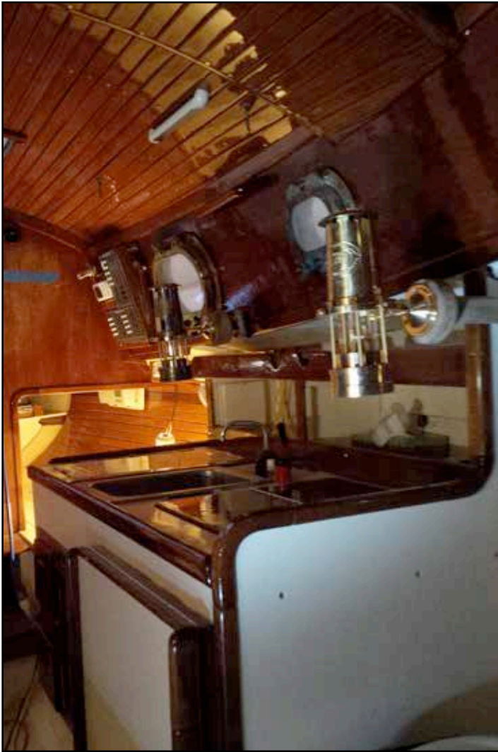
Work is nearly done in the galley. Photo: Ian Williams © 2013
