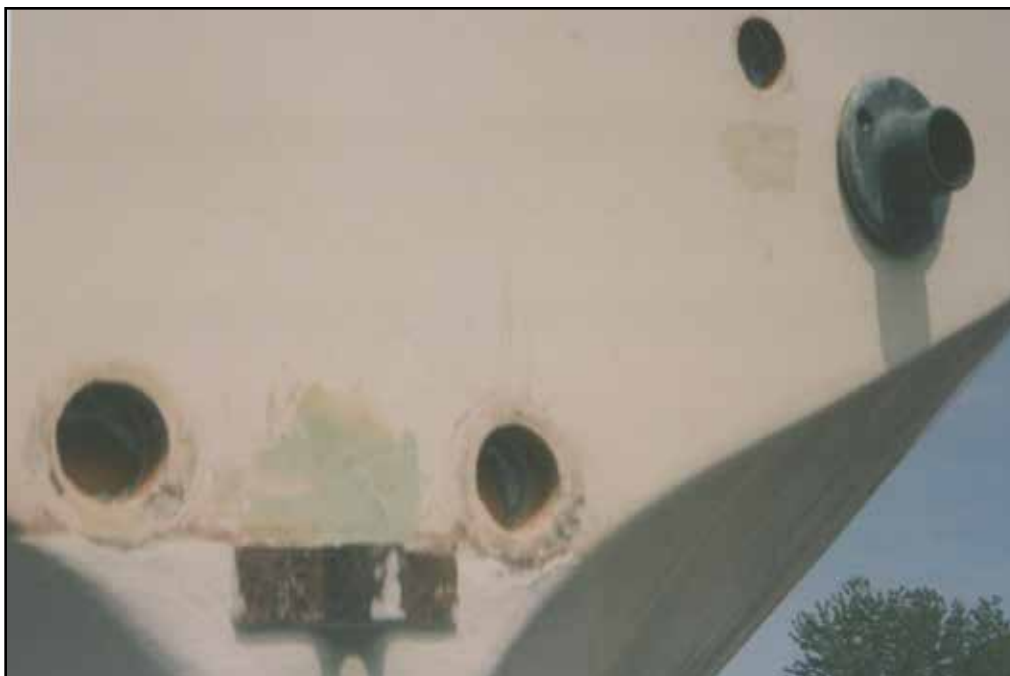
The old cockpit drains and another hole were sealed. Photo: Ian Williams © 2013
