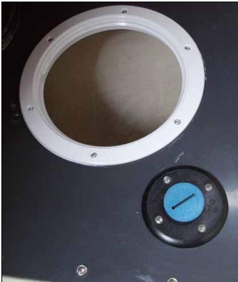
The new inspection port in place. Photo: Daryl Clark © 2013
