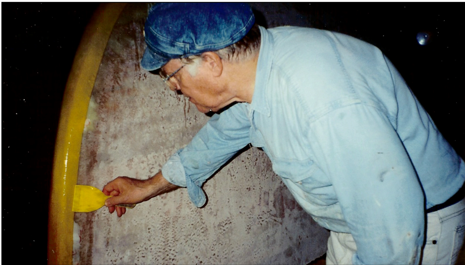
A layer of kevlar was added from stem to stern in case of grounding. Photo: Bob Collier © 2013
