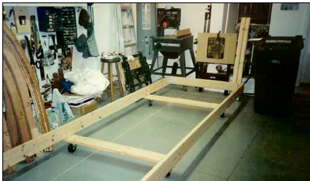
The building rig constructed. The frames were then attached to it by cross members of 2x4's. The rolling jib was a great idea.
