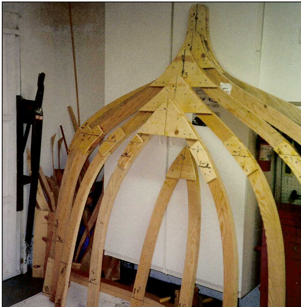
Half of the frames have been completed. For added strength, the gussets were added in front and back of the frame.
