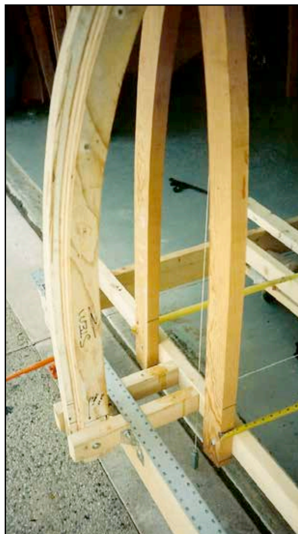
Using jacks and a plumb bob for centering.
