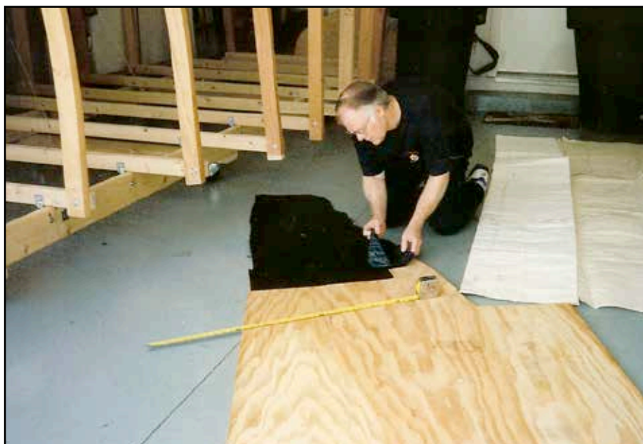
Carbon copying for the deadwood (that area of wood or fiberglass between the transom and the keel. It provides support for the motor shaft, the shaft log). You also see the frames attached to the building jig.
