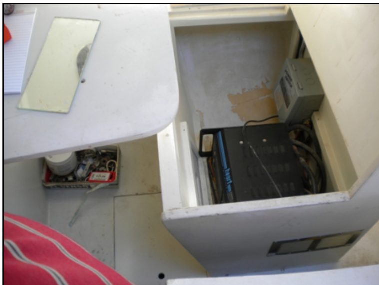
Power supply moved into closet and AC in place. Photo: Bill Cartwright © 2013
