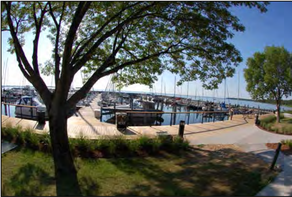
A new boardwalk was installed in 2012. Photo: Tom Davison © 2013
