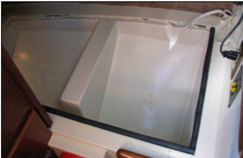
Placing the new gasket material into the edge of the tank. Photo: Dick Behan © 2013
