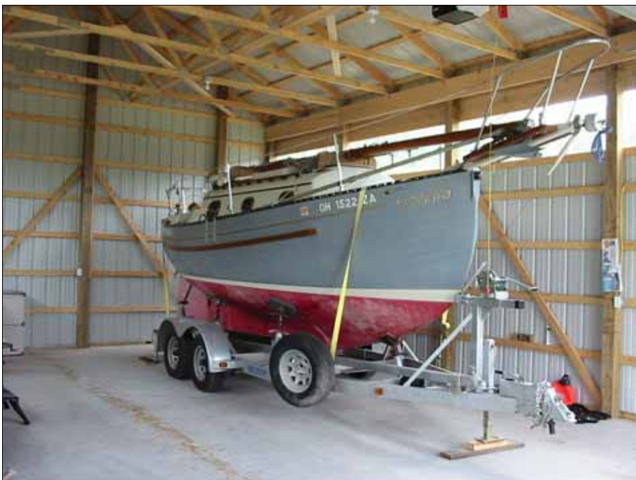
The floor is rated for 10,000 pounds per square foot, more than enough for the Flicka and trailer.
