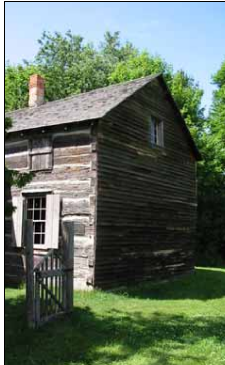
The east wall of the house shows the siding used to dress up an old log house.
