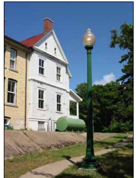
The addition was built differently from the lighthouse and adjoining keepers quarters.
