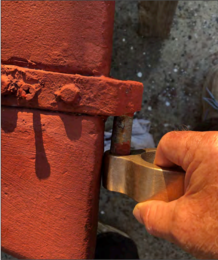
Test fitting of the new gudgeon. Photo: Jamie White © 2020
