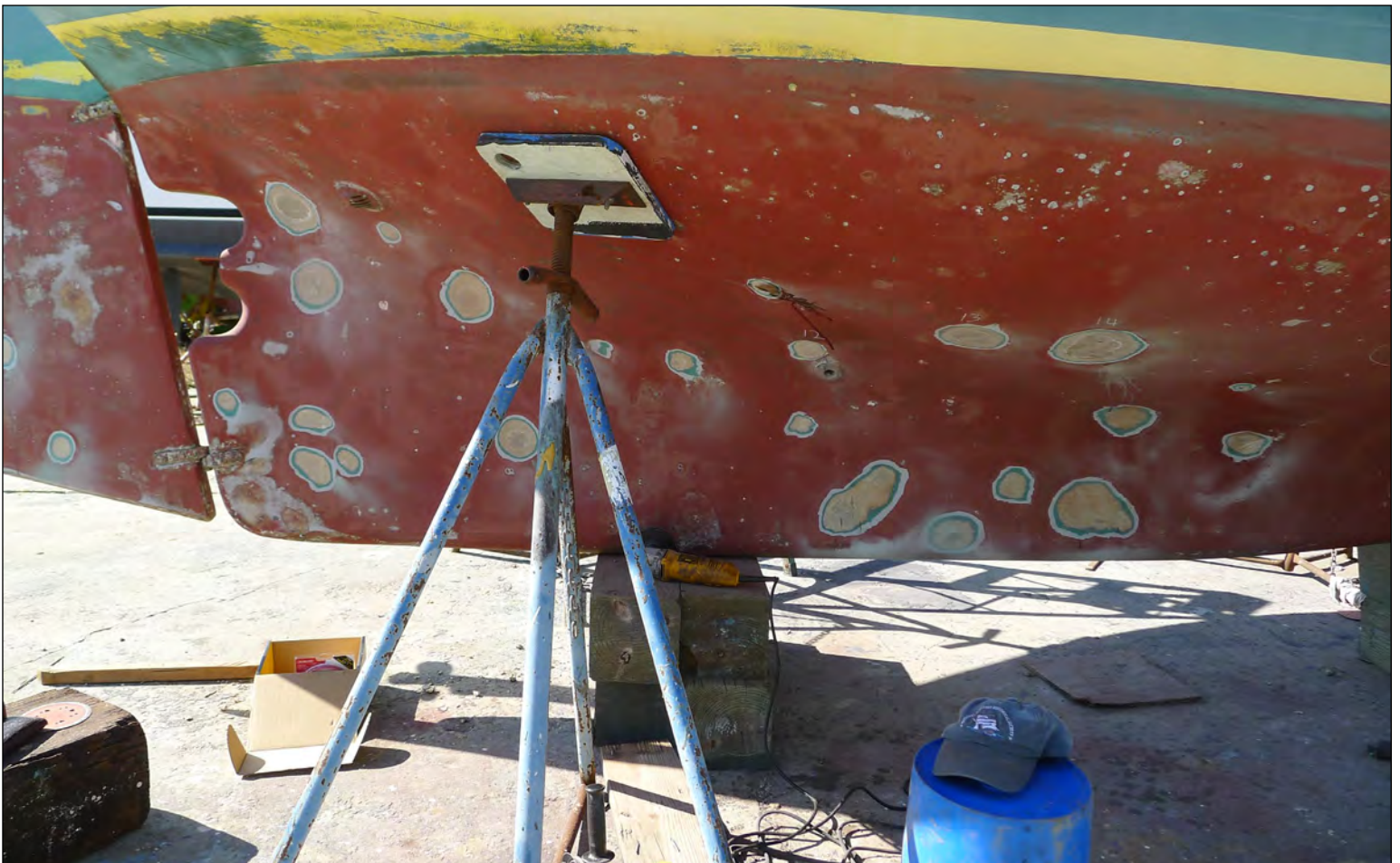
Starboard side ground down – next step finish port side and start laying up fiberglass cloth. Photo: Jamie White © 2020
