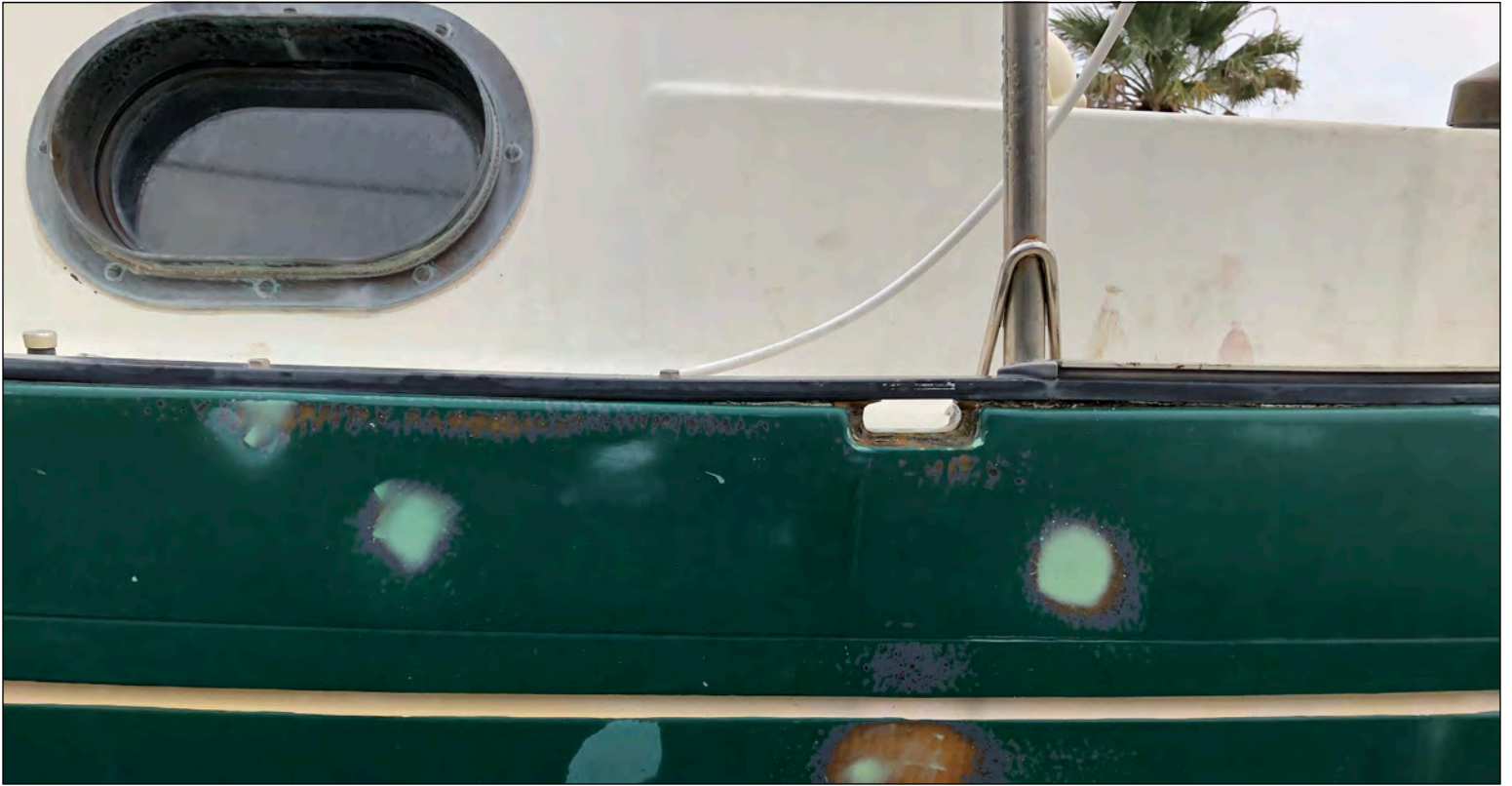
Port deck seam and various repairs including the port scupper. Photo: Jamie White © 2020
