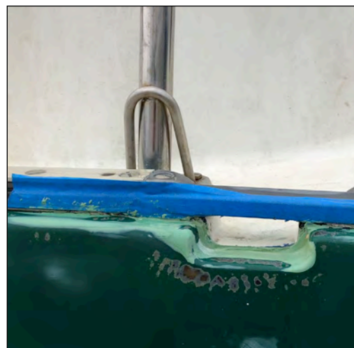
Repair to starboard scupper using strips of fiberglass cloth under two-part epoxy filler and fairing compound by Total Boat . I highly recommend it Photo: Jamie White © 2020
