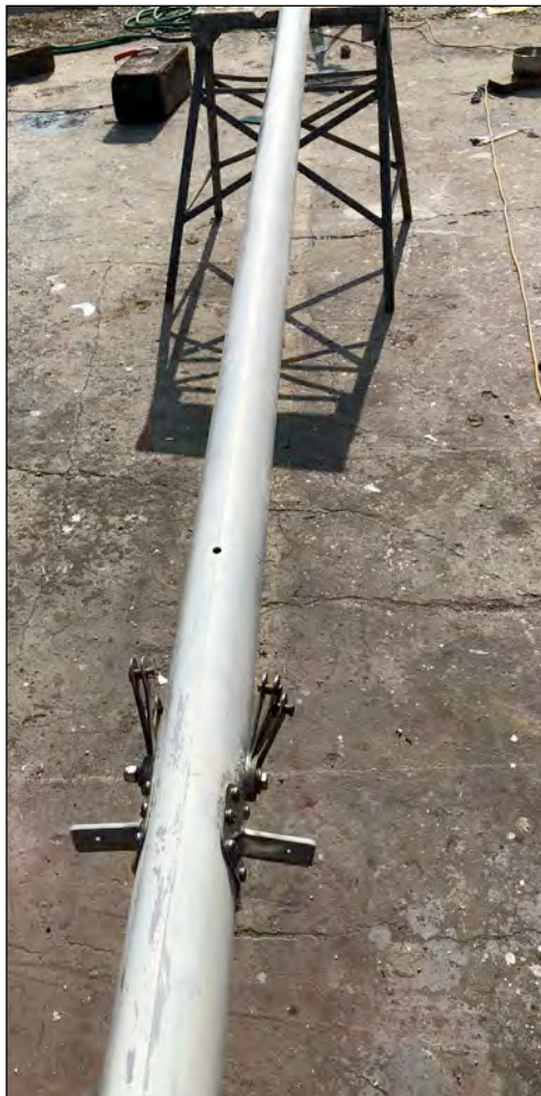
Removing paint and oxidation with a combination of chemical strippers and soft abrading wheels on an electric drill. Photo: Jamie White © 2020
