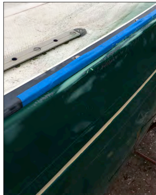
Hull repair along the hull/deck seam. Photo: Jamie White © 2020
