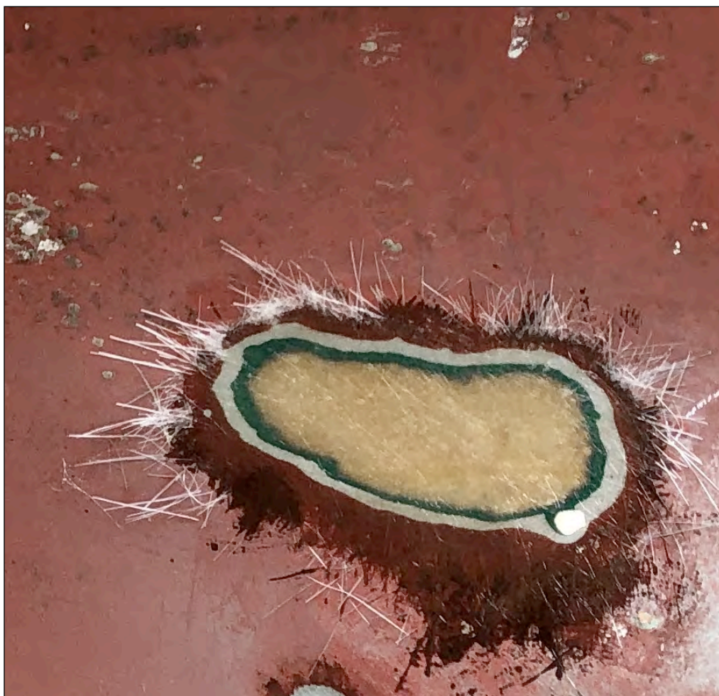
The needle-like ends of the cured fiberglass are easily sanded down.
