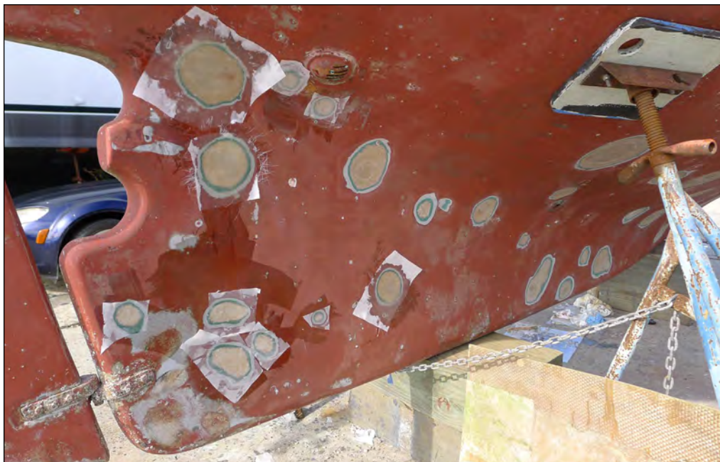
Peel-Ply on the starboard side bister repairs. Photo: Jamie White © 2020
