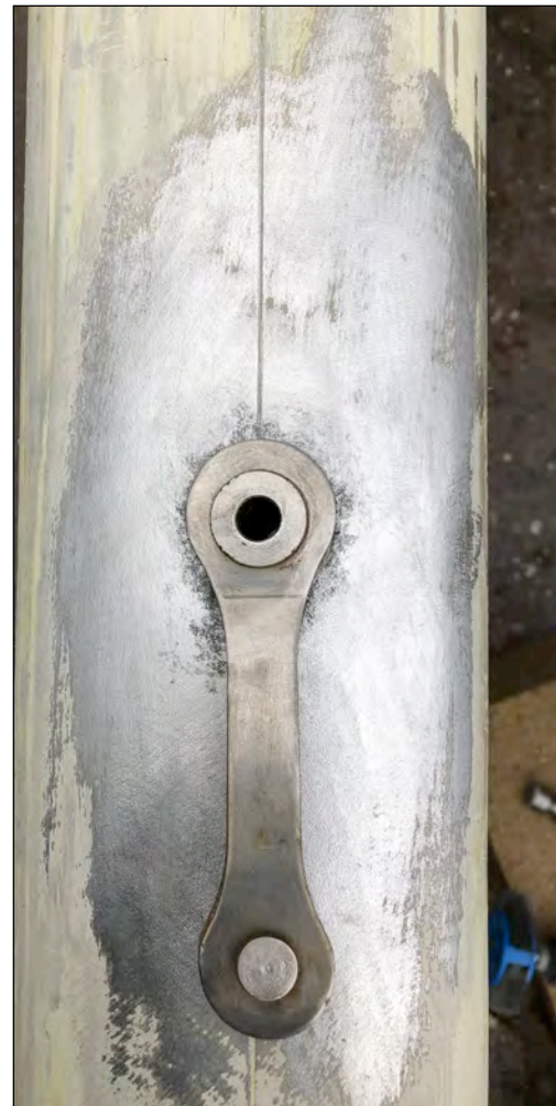
After doing a dye-pen test of the tangs, I decided to not remove them at this haul-out, as they showed no fissures or cracks. Photo: Jamie White © 2020
