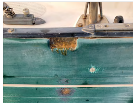
The previous repair to the port scupper. Photo: Jamie White © 2020
