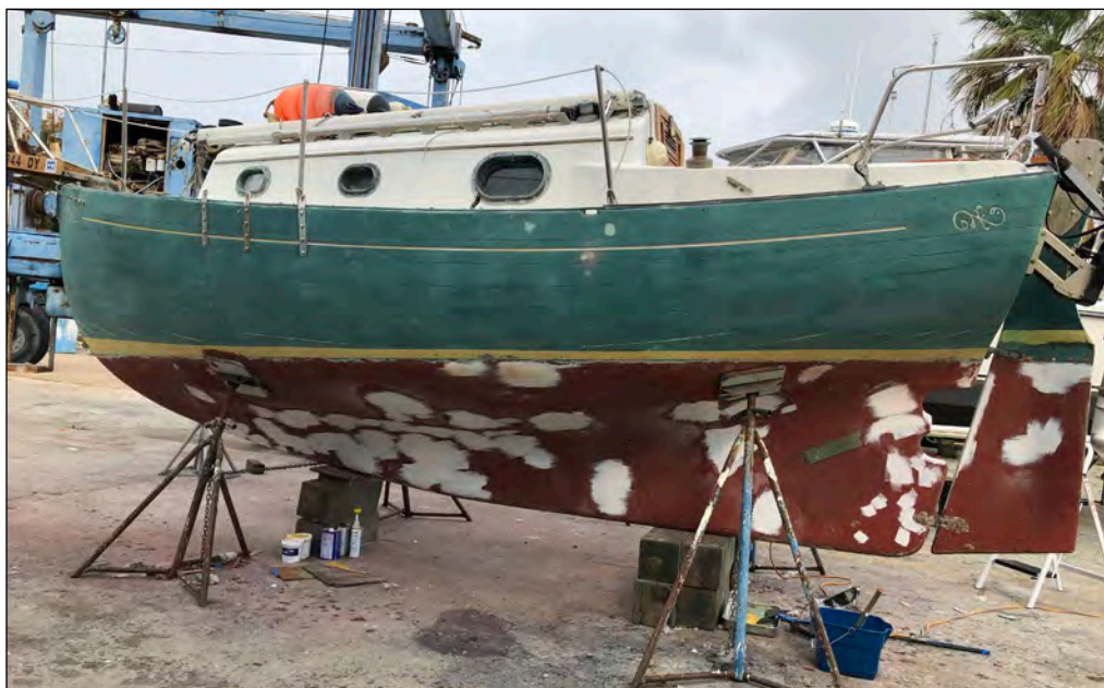
The repaired areas were covered with four coats of barrier coat. Photo: Jamie White © 2020
