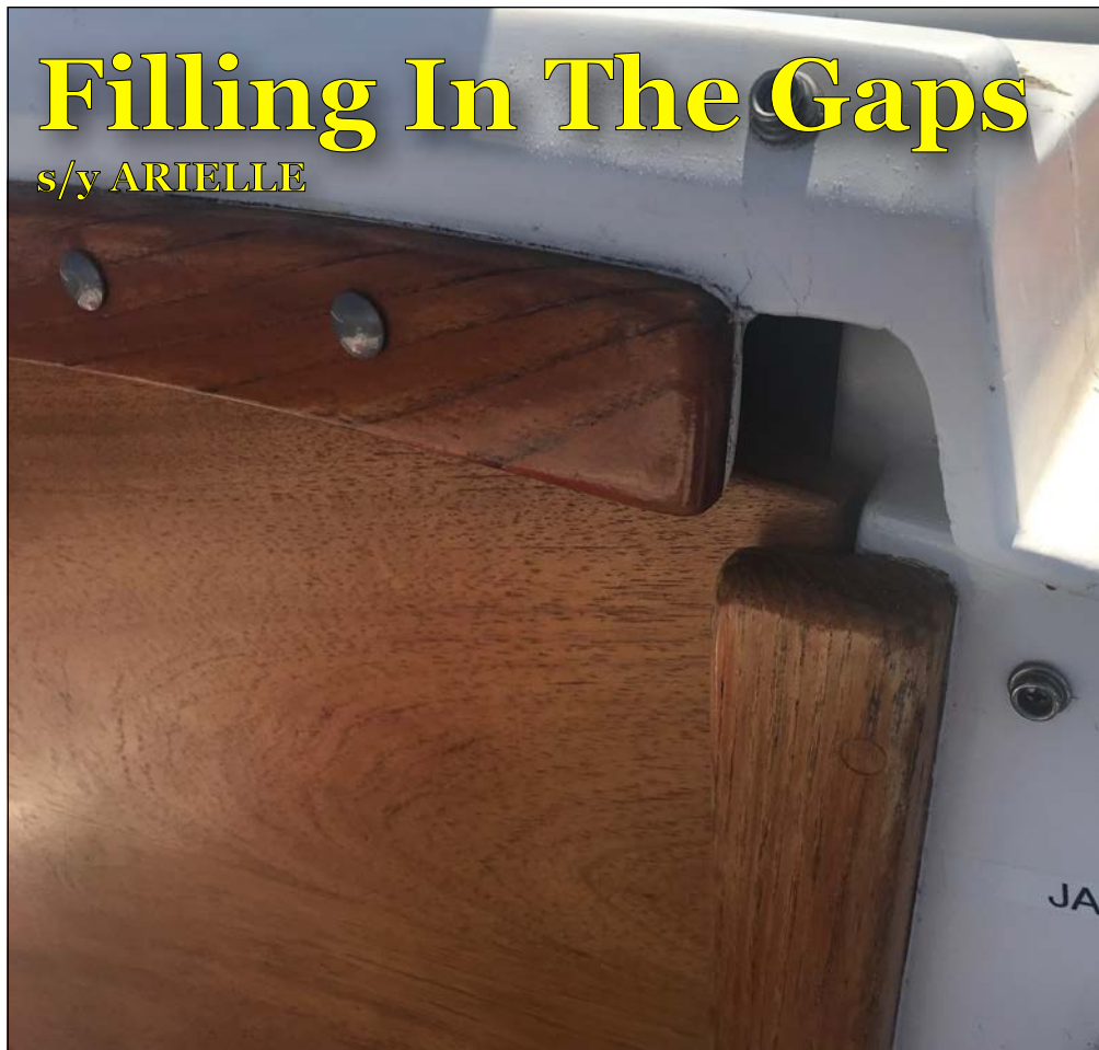
The gap in the companionway that allowed rain to enter.
