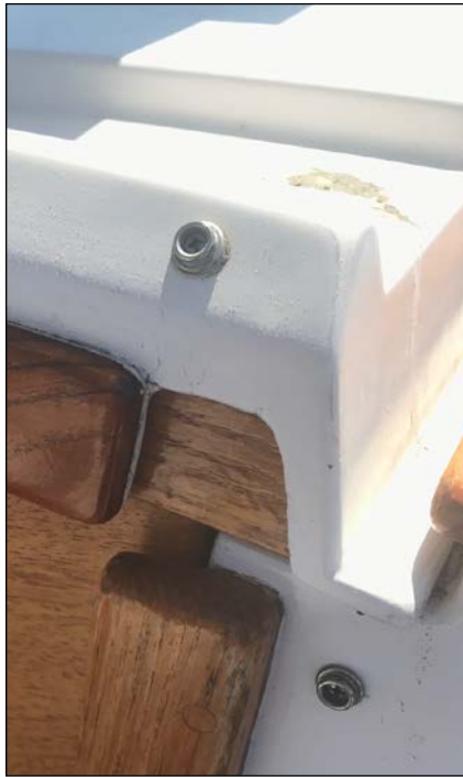
The gap is now filled Photo: Jack Russell © 2020
