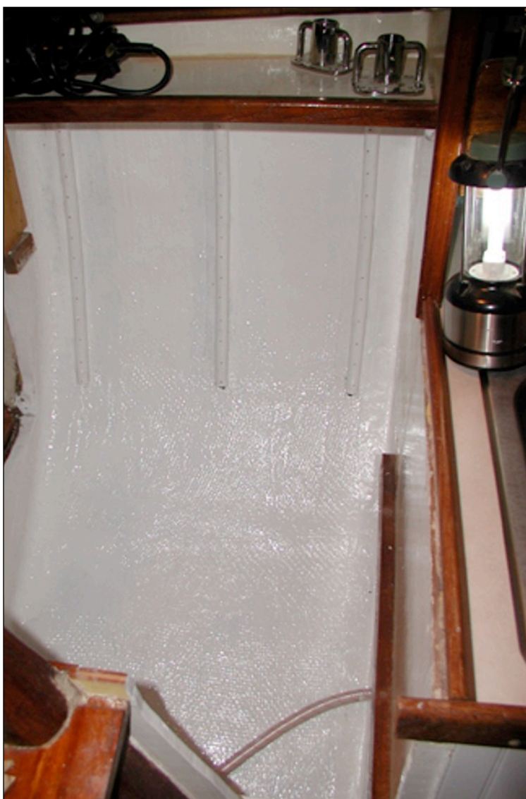
PVC pipes, heated, formed, and fiberglassed to the hull for installing the mahogany ceiling. Photo: Debbie & Jim Custer © 2020
