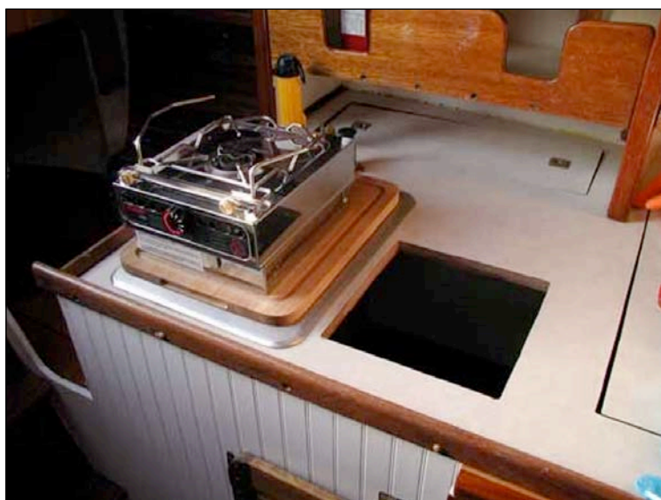
Installing the new Origo alcohol stove. Photo: Debbie & Jim Custer © 2020
