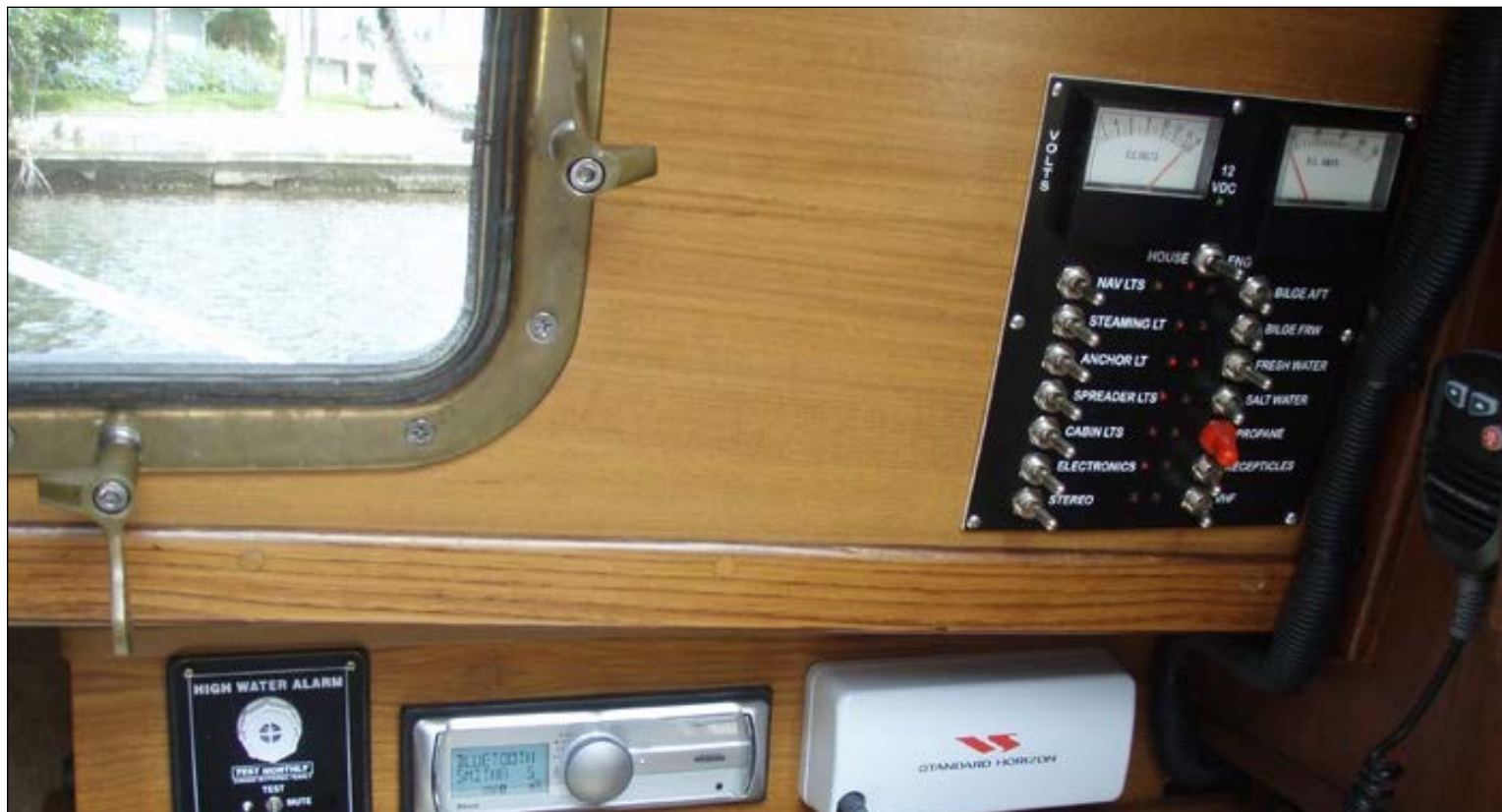
The electrical panel, stereo, and radio installation aboard s/ y MIRA JANE . Photo: Lynne Silva © 2020
